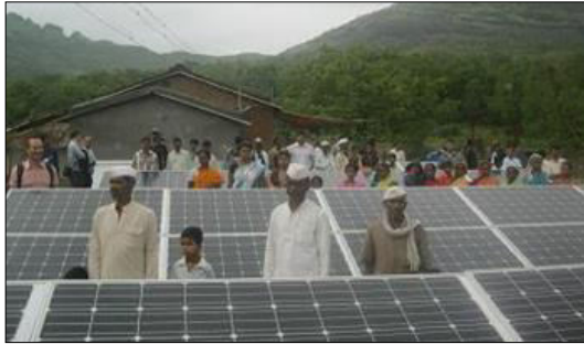
Solar PV Microgrid System at Darewadi
