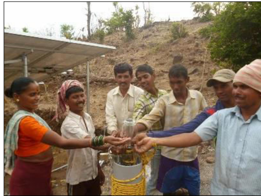
Solar Pumps at Jawhar, Palghar
